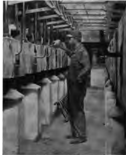
Fig. 4. Extension Oil Pipes, on Wire Drawing Frame.*
